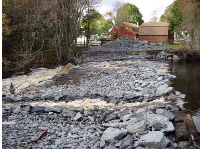
Temporary rock dam constructed immediately downstream of original dam.
