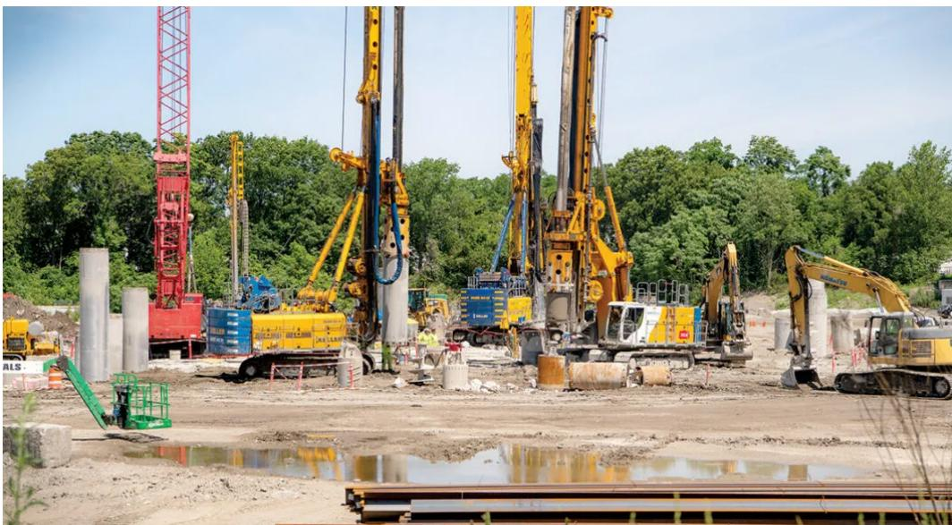
*DIGGING IT: Workers for the contractor CB3A start working on the main shaft of the combined sewer overflow tunnel that will run more than 100 feet below the city of Pawtucket. The shaft, located on School Street in Pawtucket, will be 60 feet in diameter and will allow a boring machine to be lowered in. / COURTESY NARRAGANSETT BAY COMMISSION/PETER GOLDBERG*
